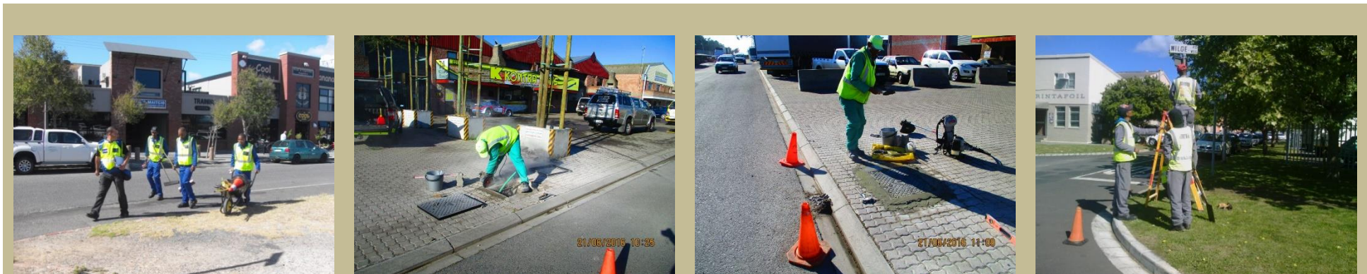
Figure 18 the combination of social upliftment through job creation and the development of an urban maintenance team have had positive results in other SRAs
