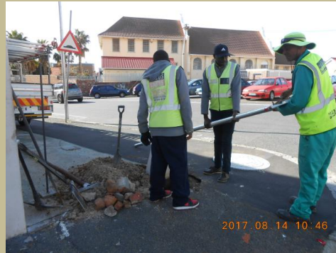
Previously homeless men living at a shelter repairs public infrastructure in the SRBID
