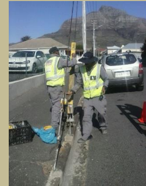
A maintenance team comprising of workers from an NGO working with homeless people provide painters to beautify the area
