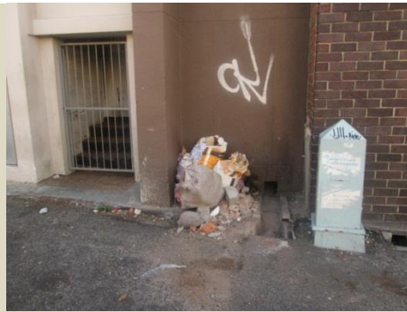
Figure 12 Evidence of illegal dumping – in this case house hold waste and builder's rubble
