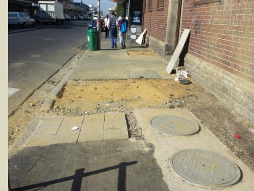
Figure 19 Broken manhole covers on sidewalks
