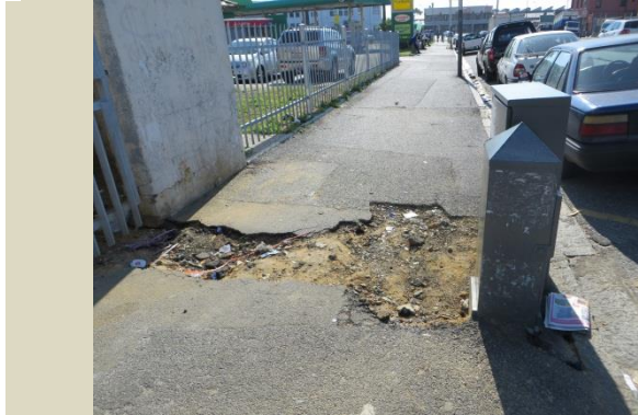
Figure 18 Unmaintained sidewalk surfaces
