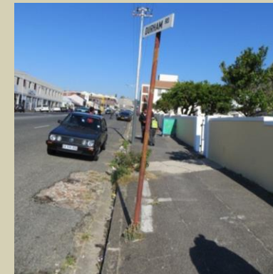
Figure 16 Poor quality of street and information signs
