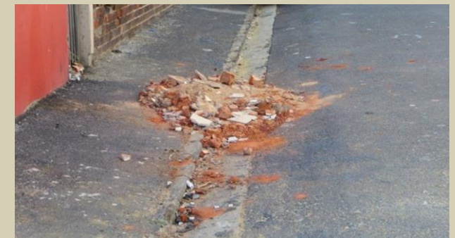
Figure 9 Illegal dumping of builders rubble
